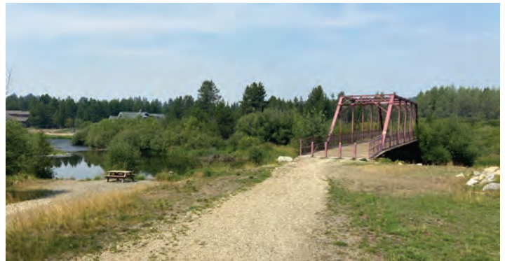
Sheep Bridge and Existing River Access
